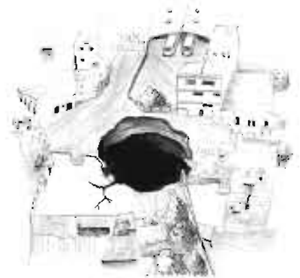
sinkhole in Guatemala City caused by a burst sewer drawing into the base volcanic pumice bedrock
