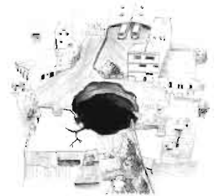
sinkhole in Guatemala City caused by a burst sewer draining into the base volcanic pumice bedrock
